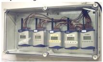
Alarms are incorporated into the system and have been configured to automatically send SMS text messages from the logger to Morgan, who can then check the system status and decide what course of action to follow. This installation also includes excess CO2 and O2 depletion alarms for laboratories where there is piped CO2.
